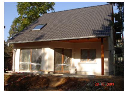
Bauvorhaben in Chemnitz
